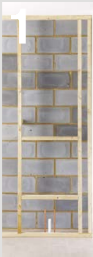
01 Install timber-frame (supplied by others).
