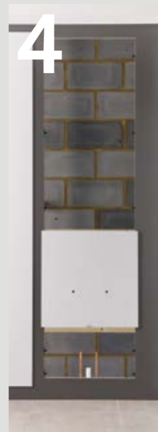
04 Drill or cut out for sanitaryware.
