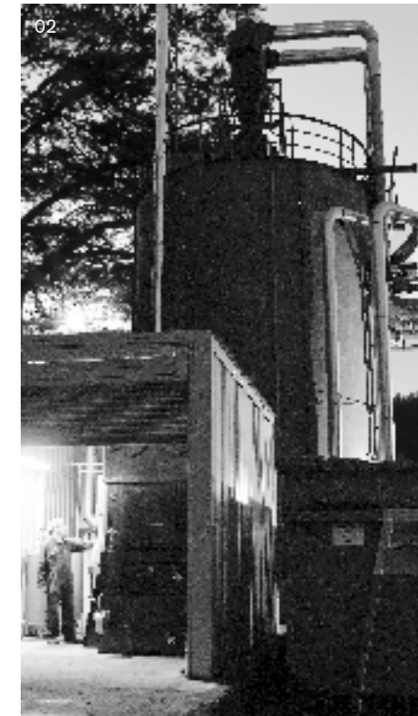
01-02 Waste management Biomass burner turns production waste into factory and office heating.
